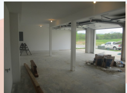
View of garage interior (photo taken during construction)
