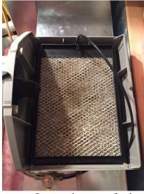
• Locate the water feeder tube at the top of the humidifier pad:
