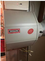
Remove the lid of the humidifier. It should lift up and off and there should be instructions on it to guide you. Once you remove the lid, you will be able to see the humidifier pad like this:
